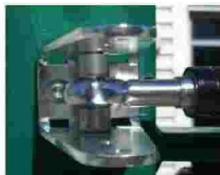
Post bracket with spacers and gate closer attached
